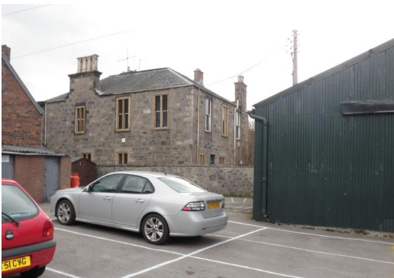
Photo 3 Side Elevation to Car Park as Existing
